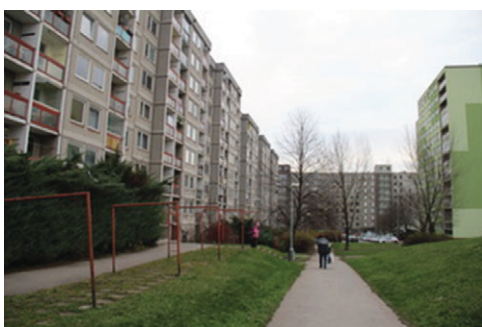
Figure 7 Prague, Cerny Most housing estate, 2015 (source: author)
