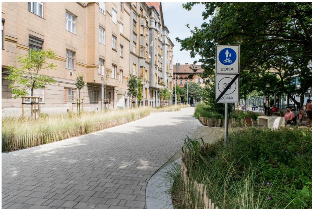
Picture HU4. Changing a street into multifunctional pedestrian green area, Déri Miksa utca, Budapest 8th District, 2022. 3-storey vegetation, semi-permeable pavements and resting places were developed. (Photo Credit: www.jozsefvaros.hu )
